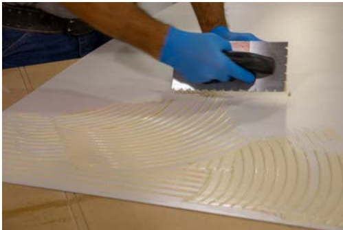
Apply adhesive. 100% adhesive coverage required.
