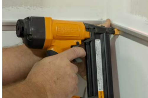
16-18 gauge 1" nails used to hold trim
