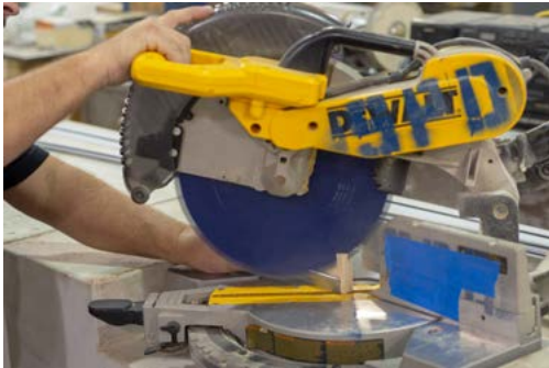
Cut trim & miter corners
